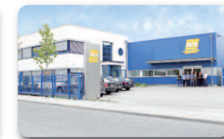
RINGSPANN RCS GmbH, Germany Plant Remote Control Systems
